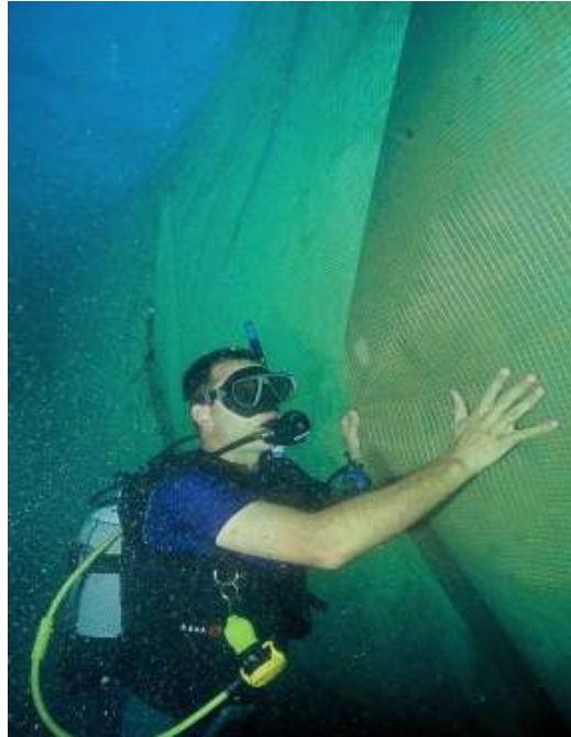
Figure 15 – Installation of Silt Curtains
